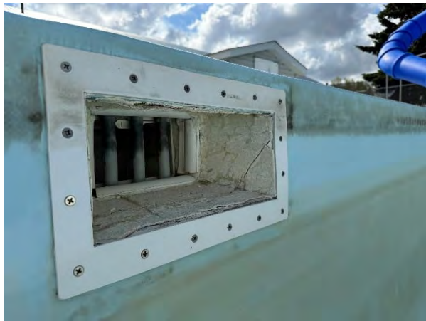
Figure 8- Cracked Skimmer
