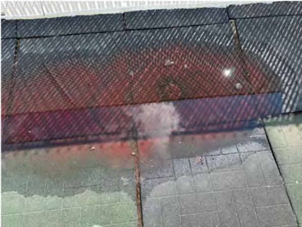
Figure 3 - Poor Drainage
