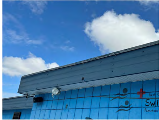
Figure 14 - Damaged Flashing
