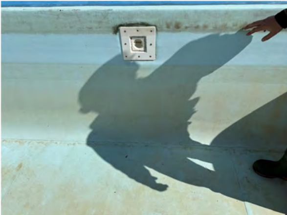
Figure 9 – Stained Vinyl Liner
