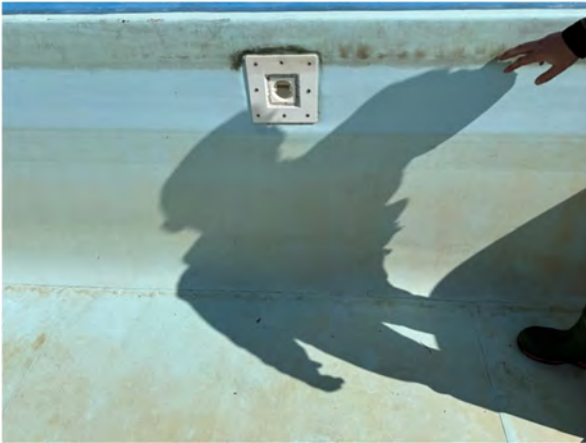
Figure 5 – Stained Vinyl Liner
